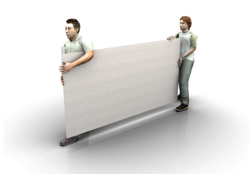
Figure 3 Always carry the panel on edge but DO NOT store on edge
