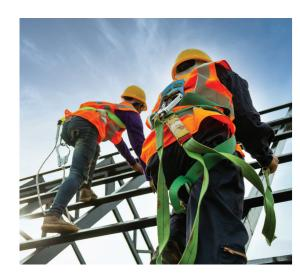
Do not step on the Eter sheet during installation or service. Stepping or walking directly on the Ether roofing may cause cracks in the product and or lead to work accidents.
